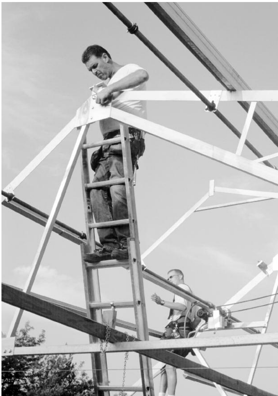
Steve Hopper, left, and Greg Veasman of Hummert International prepare to put a new roof of rigid clear plastic on our greenhouse, after removing a 14-year-old flexible sheeting roof that had weathered to tattering.
