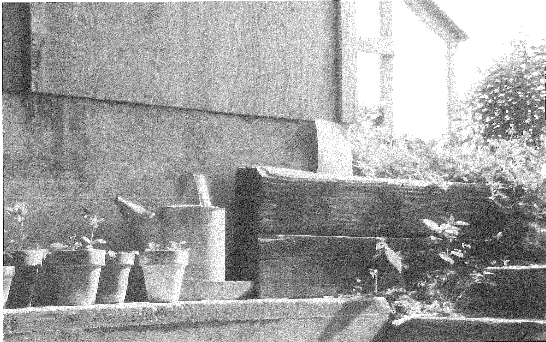
Southeast side of classroom building at The Land
