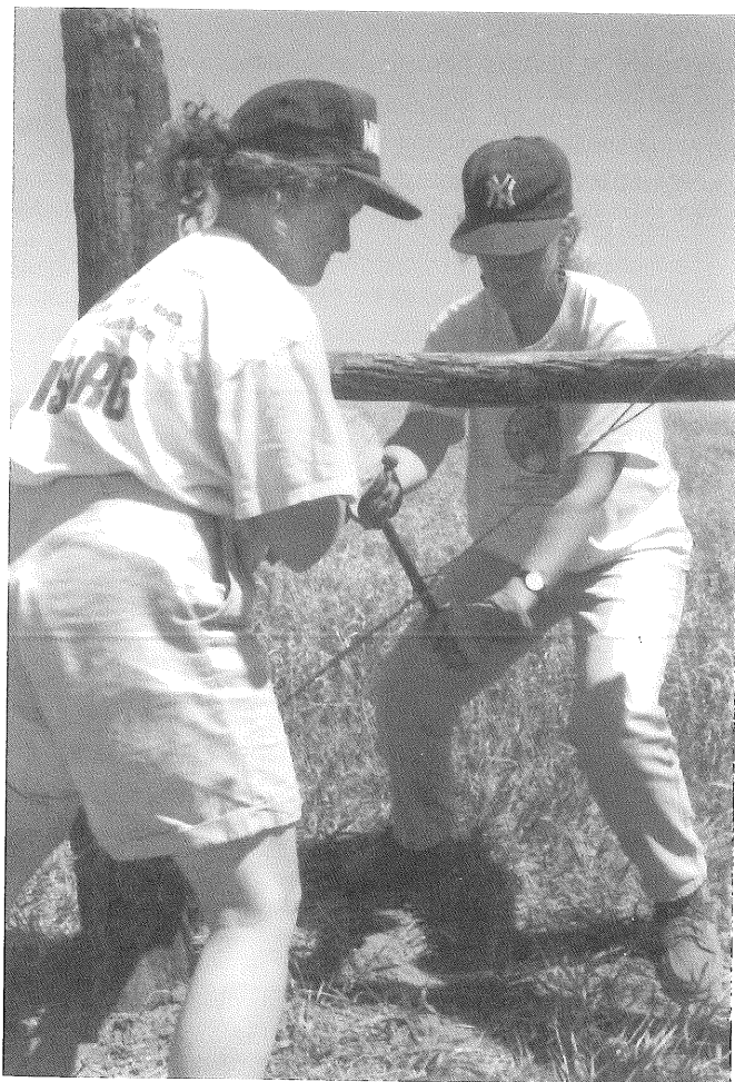
1994 interns Portia Blume and Kathy Holm building fence
