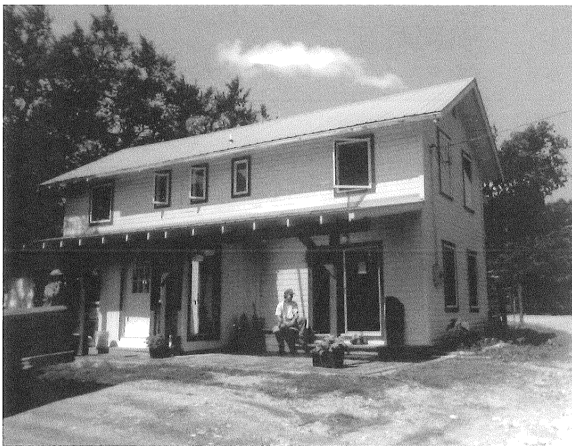
The renovated hardware store building in Matfield Green
