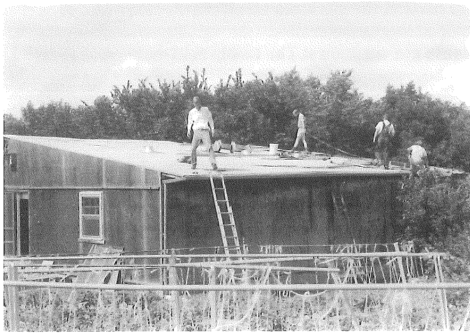
Repairing the classroom roof after the 1987 storm
