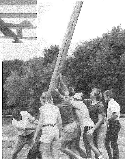
Raising the barn poles
