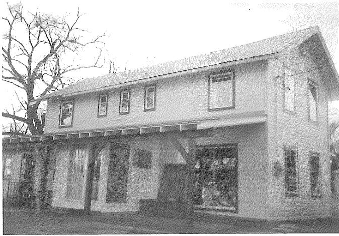
The remodeled "Lumberyard Cafe" in Matfield Green
