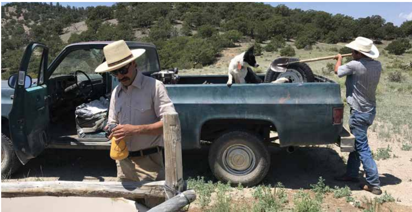
Sam and a colleague fix a float valve on a cattle tank. Photo by Taylor Muglia.
