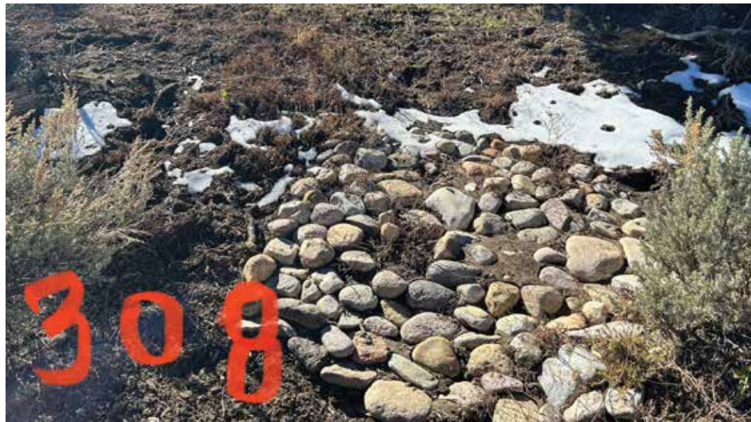
A compost plot (number 308) uphill of the erosion control structure holding snow. Rock run-downs are particularly useful in erosion zones where headcuts, or a zone of steep, quick elevation changes cause water to move more rapidly downstream. By building ramp-like structures with stones, we can slow the movement of water through and reduce erosion. Note also the extent that silt has already accumulated in parts of the rock structure indicating that soil is held high on the land and not sloughing off downstream. Check out Quivira's erosion control technical guide for details.
