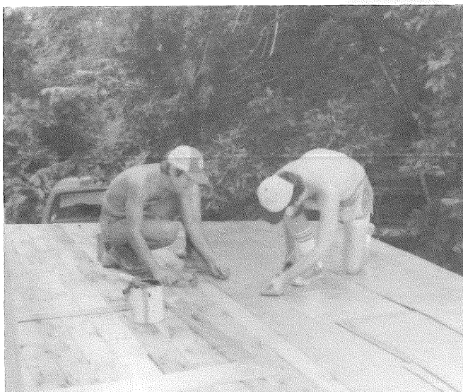
Paul Rasch & Mark Bigelow roofing the saw shed.
