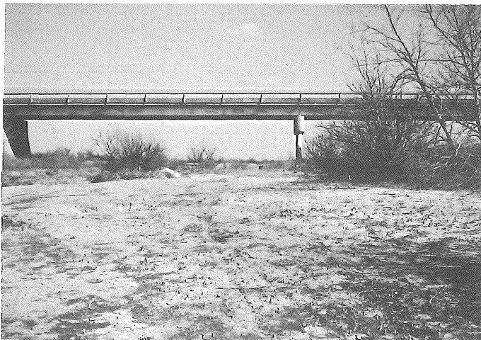
The Arkansas River Bed at Holcomb
