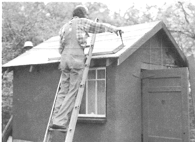
Paul Krumm, operations manager, installs the photovoltaic panel on composting toilet.
