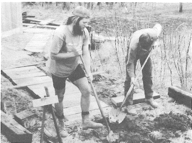
Mark S. and Patrick B. build new boardwalk.
