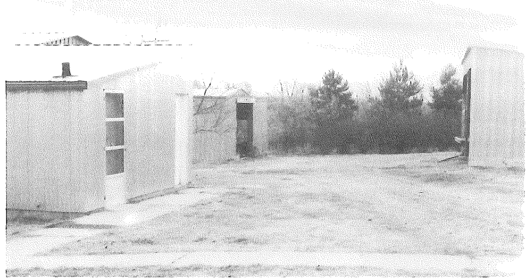
Left, building attached to shop (shop roof upper left). Center, storage barn. Right, pole shed.
