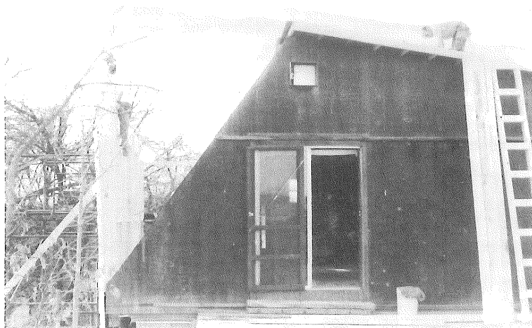
A new south wall is started.
