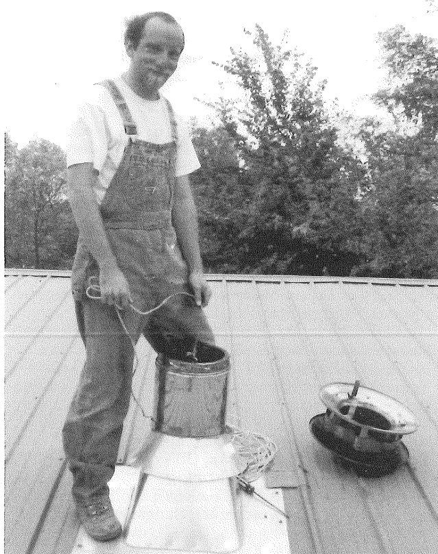
Darryl Short cleans the classroom chimneys.
