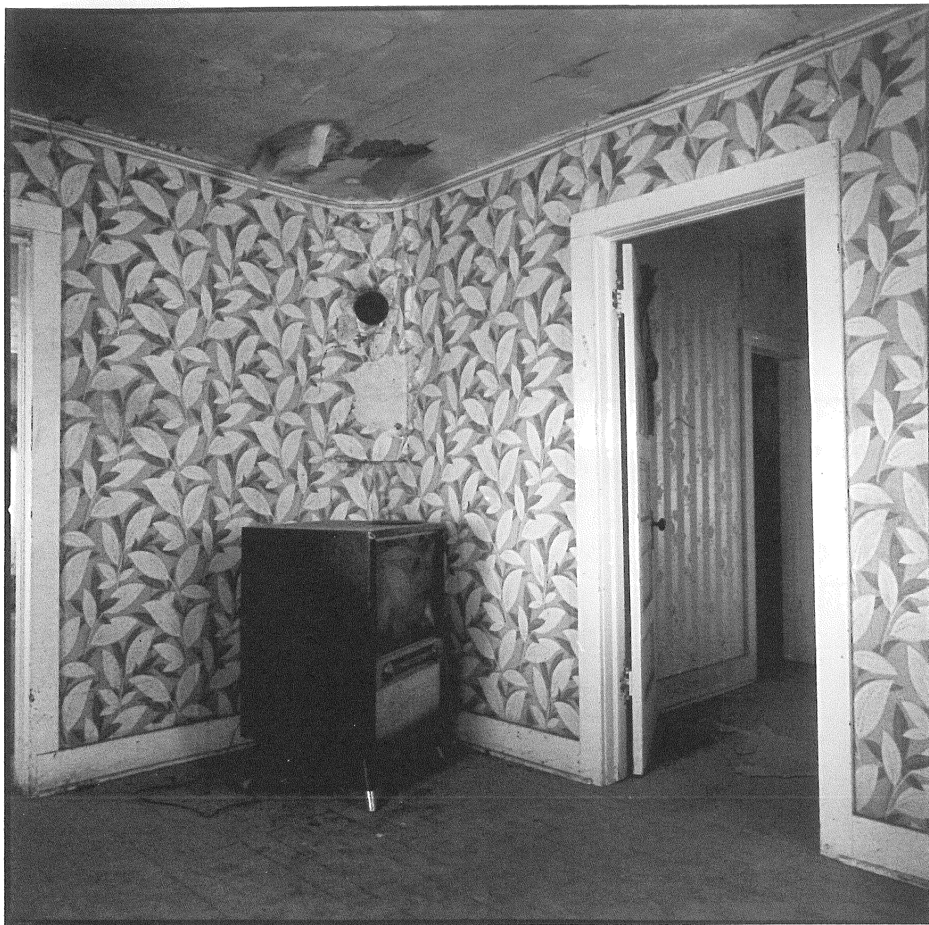
Abandoned house, August 17, 1991 — Matfield Green
