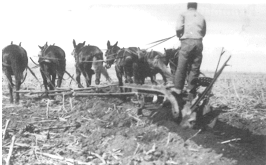
Six-mule team drawing a Corsicana eight-foot terracing machine, c. 1935.
